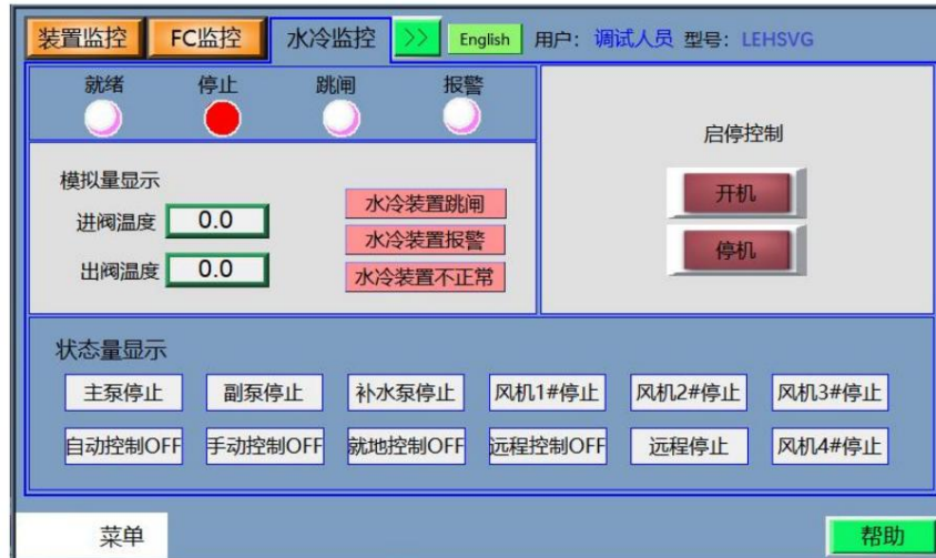
Figure 5.12 LEHSVG touch screen water cooling control interface
