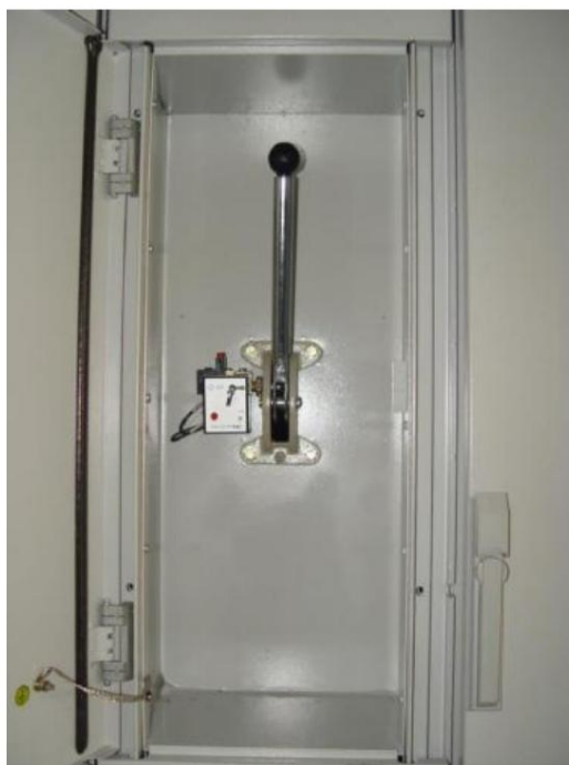
Figure 7.4 Operating lever position when the isolating switch is closed
