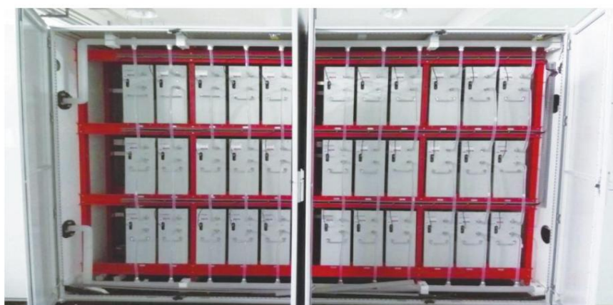
Figure 4.7 Arrangement of units in water-cooled power cabinet
