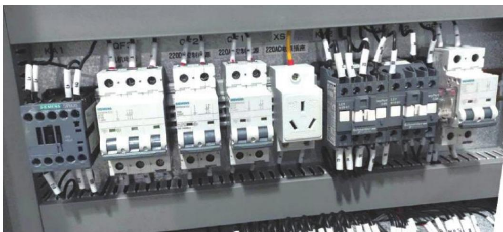
Figure 7.3 Control cabinet layout
