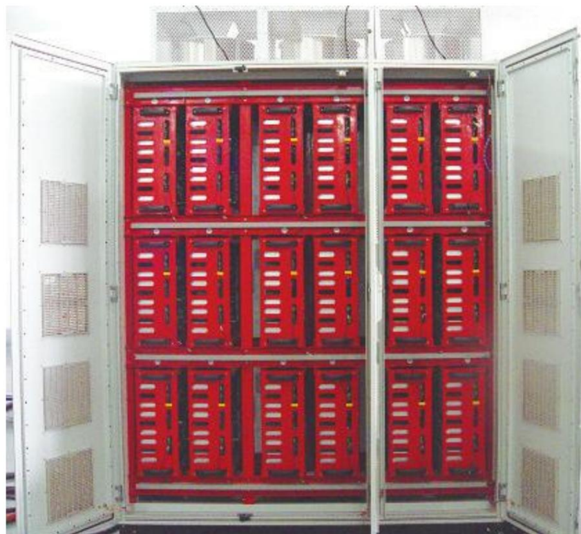
Figure 4.6 Arrangement of units in air-cooled power cabinet
